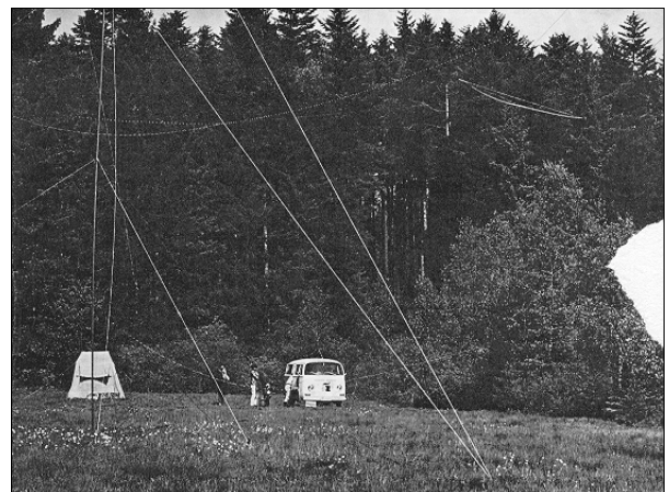
Im Hochmoor: 80m-ZL-Spezial, 40m-3 Element Yagi, 20, 15, 10m-2 Element Quad
